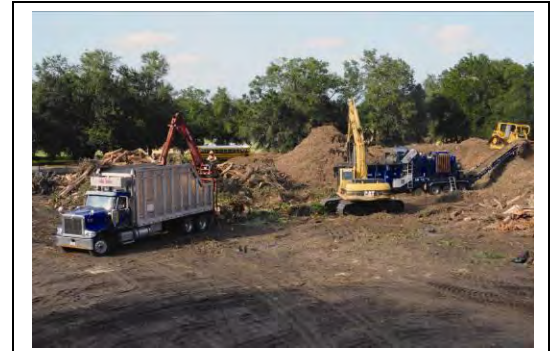
Figure 2: Type and Duration of Equipment Used Must Be Documented
