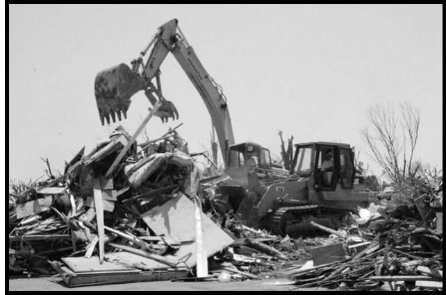
Figure 3.2 - Construction and Demolition Debris
