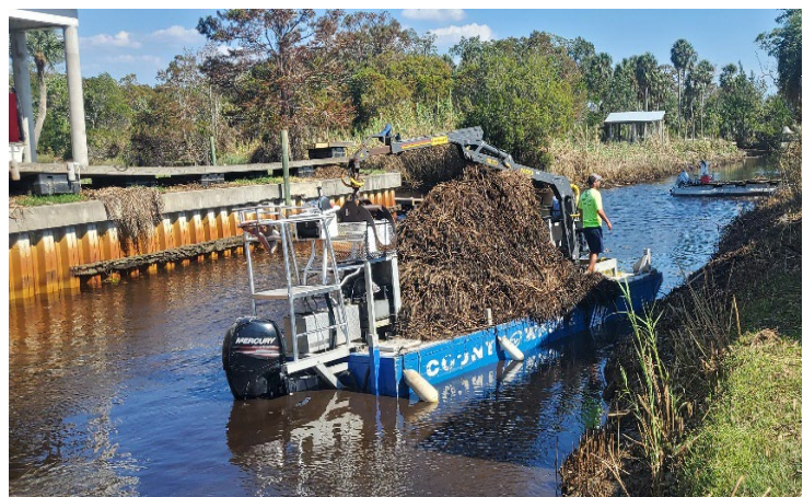
Exhibit 6. Waterway Debris Removal following Hurricane Idalia
