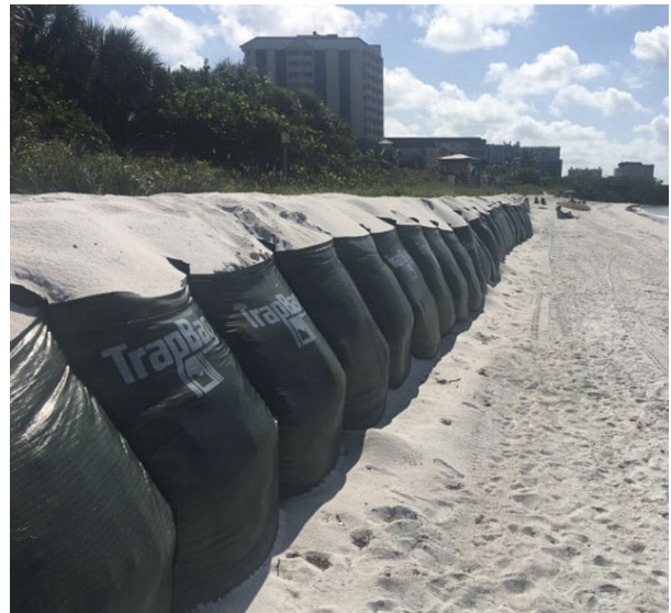
Exhibit 7. Trap Bag Installation in Volusia County, FL
